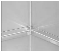
Detail of radius corner and tanked bottom
