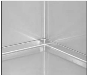
Detail of radius corner and tanked bottom
